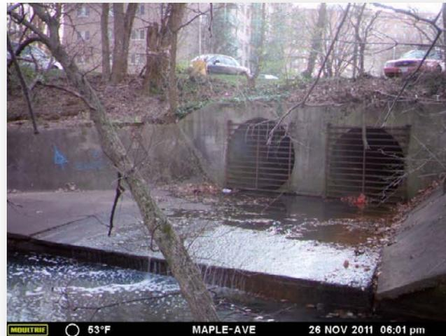
The time lapse pictures have also revealed events we would have otherwise missed, including a large discharge of sediment and/or iron algae from the right outfall pipe that covered the apron and filled the receiving pool for much of a day.
